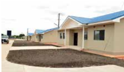
PHOTO: Police Housing Camp in Chelstone
